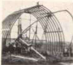
BARN UNDER CONSTRUCTION
